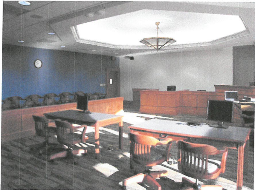
Existing features of the former Magistrate Courtroom include the judge's bench, adjacent casework, and the ceiling.
